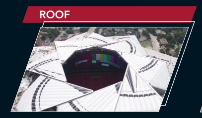
The stadium's signature feature is its retractable roof, which features a "pinwheel" consisting of eight translucent, triangular panels.
